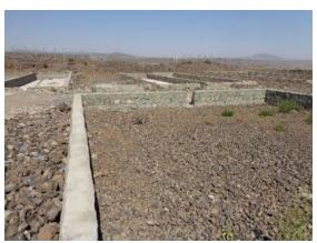
Photo: A completed Sludge Drying Bed in Welenchiti town, Oromia Region. (Photo by UNICEF, May 2017)
